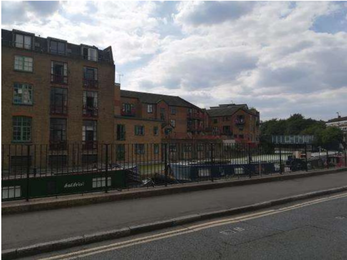
Existing site looking south west
