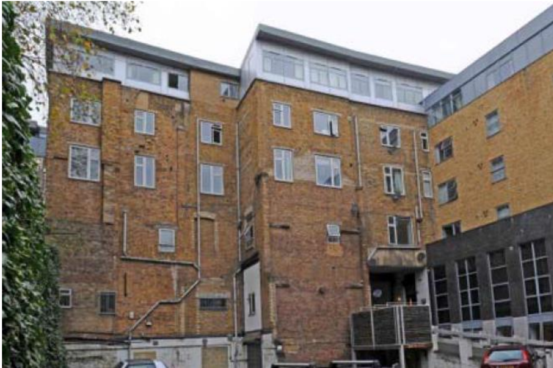
Rear of Walker House from car park
