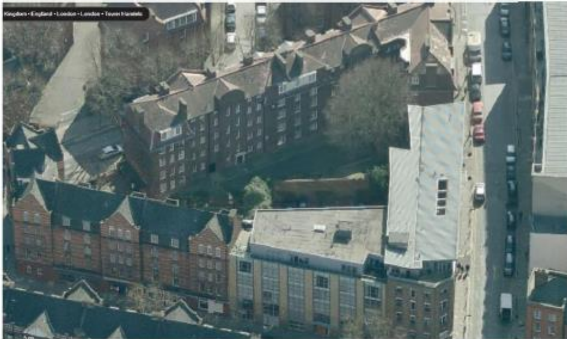
01 Aerial View from North 002
