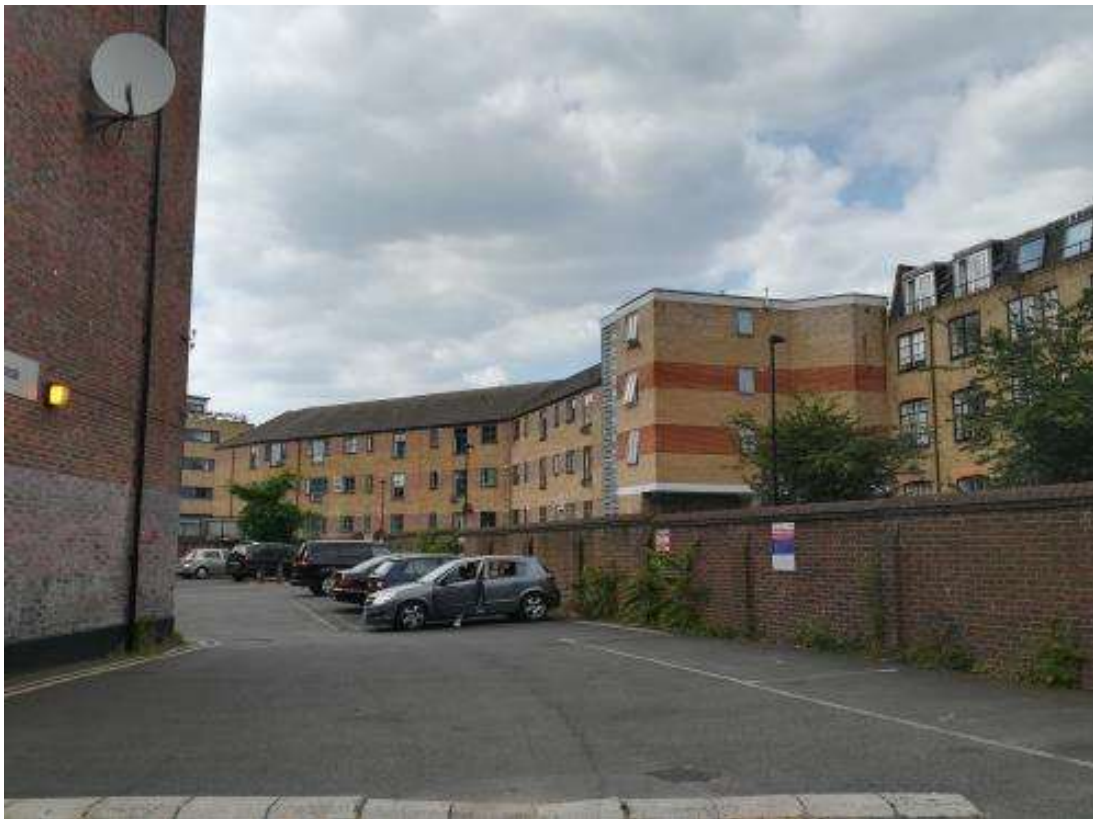
Existing site looking north east
