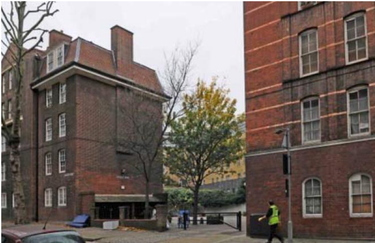
View from junction of Navarre Street, application site in background within courtyard
