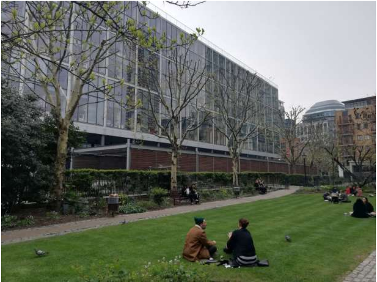
Image 6 – Existing Lamb Street structure (looking south-west from Elder Gardens)
